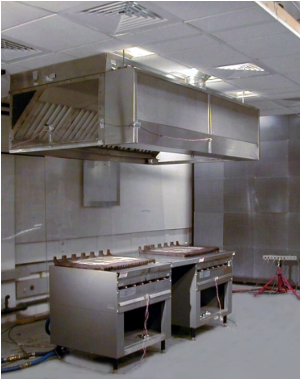
Figure 7: Two Gas Charbroilers under an 8' Hood Canopy Hood with Attached MUA Plenum with Front Face Supply
