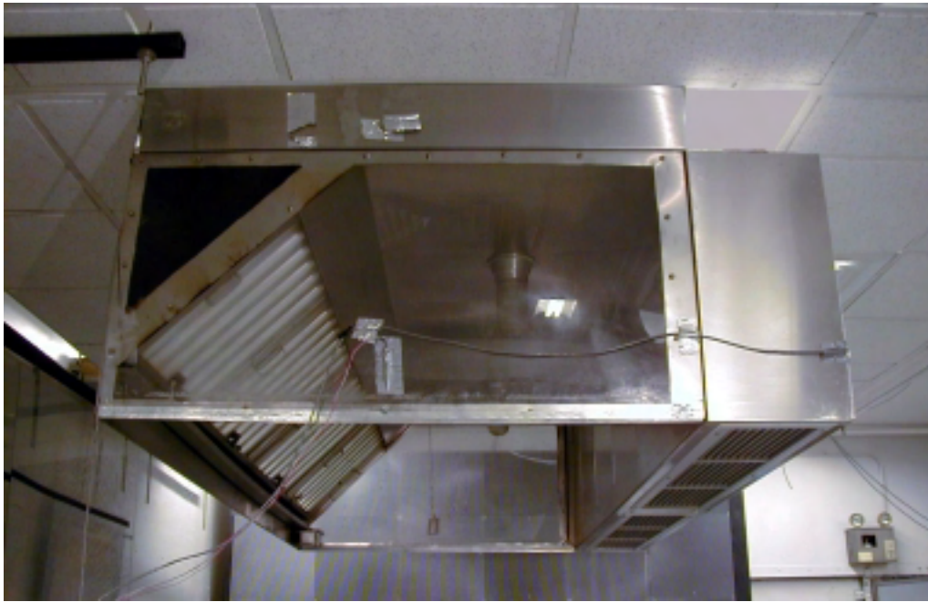
Figure 8: Side View of an 8' MUA Hood with Air Curtain Supply
